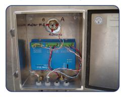
DryTrack® Metering Cards: This is where the data is processed and then sent to the control room. The meter cards are installed in aluminum NEMA 4 enclosures on the outside of the kiln walls close to each measuring point. A low-pressure air system keeps the enclosures and meter cards cool and dry by maintaining a slight positive pressure inside the meter box. This environment ensures a long life for the measuring cards and enables us to offer a 3-year warranty, the longest in the industry.
