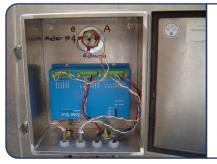
**DryTrack® Metering Cards:** This is where the data is processed and then sent to the control room. The meter cards are installed in aluminum NEMA 4 enclosures on the outside of the kiln walls close to each measuring point. A low-pressure air system keeps the enclosures and meter cards cool and dry by maintaining a slight positive pressure inside the meter box. This environment ensures a long life for the measuring cards and enables us to offer a 3-year warranty, the longest in the industry.
