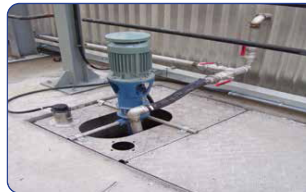
System condensate is collected and pumped back into the system for reuse.
